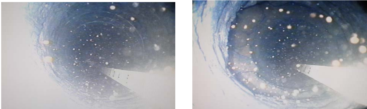
Figure 17. Screenshot from the video borehole logging showing a category 0 (left) and a category 4 (right) fracture.
